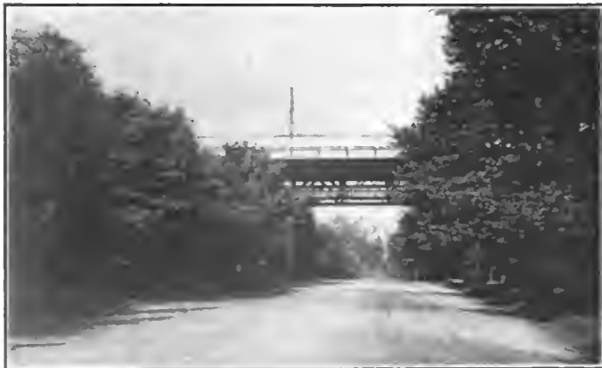
Under Strawberry Bridge on West River Drive
